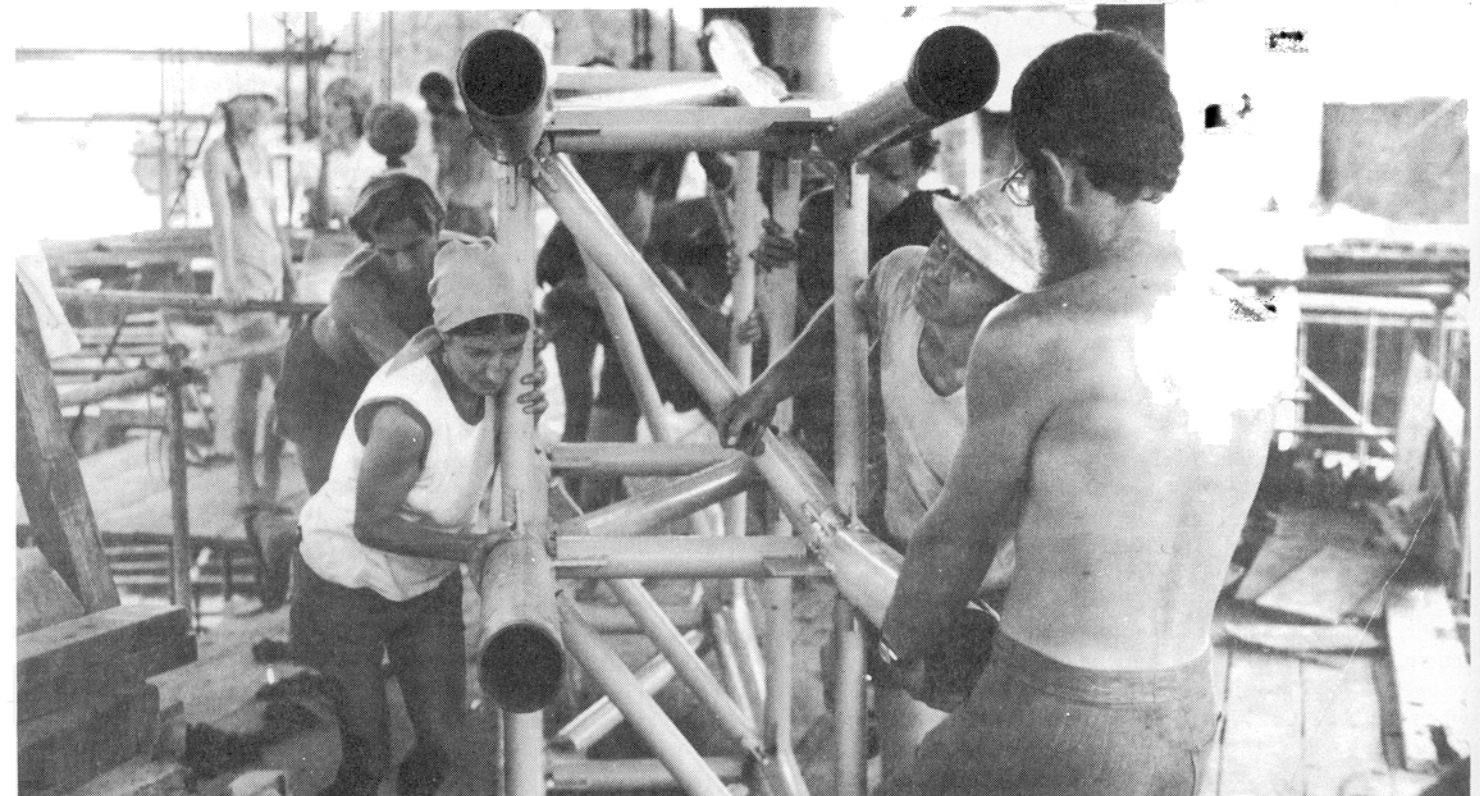
Matrimandir construction, 1979. Photo by Bill Sullivan.
